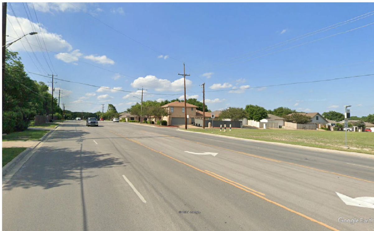
VIEW TO NORTHEAST
