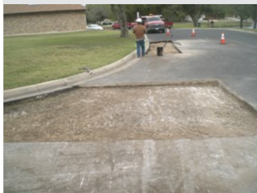
Project Photos: Point Repairs
