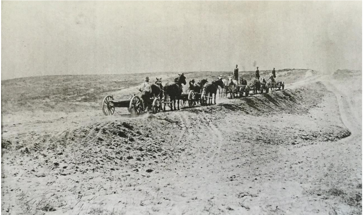
Work begins in the 1890s on the initial Perkins County canal project. (Photo courtesy of Perkins County Historical Society)
