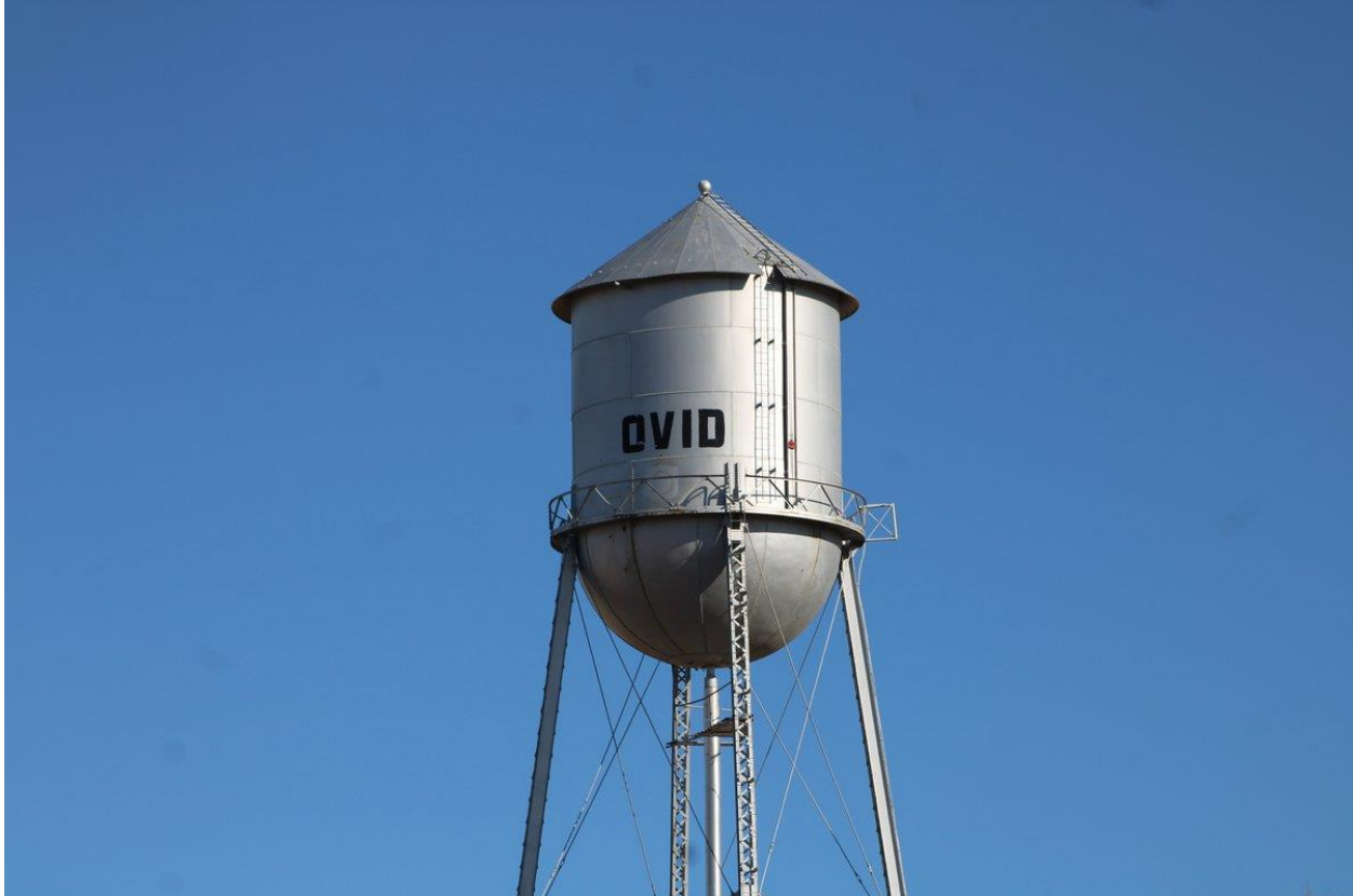
Ovid, Colorado water tank. (Photo by Fred Knapp, Nebraska Public Media News)
