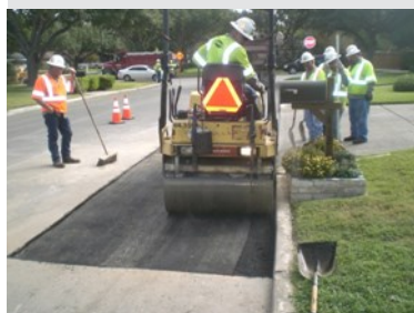
Project Photos: Point Repairs
