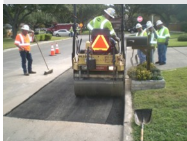
Project Photos: Point Repairs
