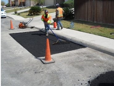
Project Photos: Point Repairs
