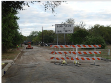
Project Photos: Parkcrest Drive
