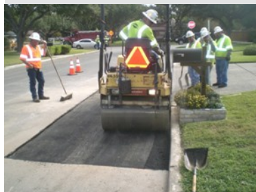
Project Photos: Point Repairs
