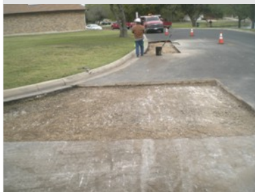
Project Photos: Point Repairs
